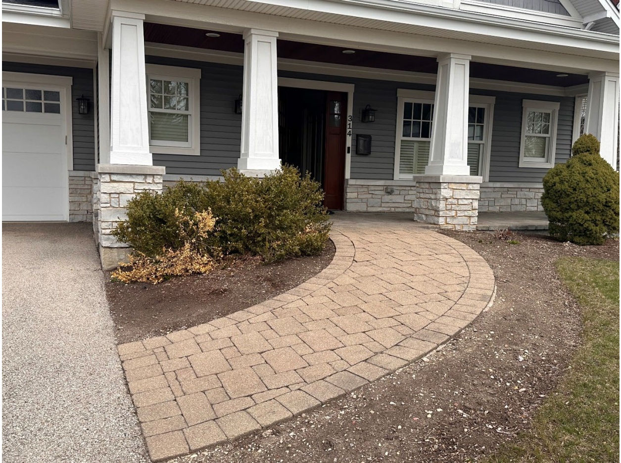
Photo 12; front walk leading up to the front door which doubles as a wheelchair ramp
