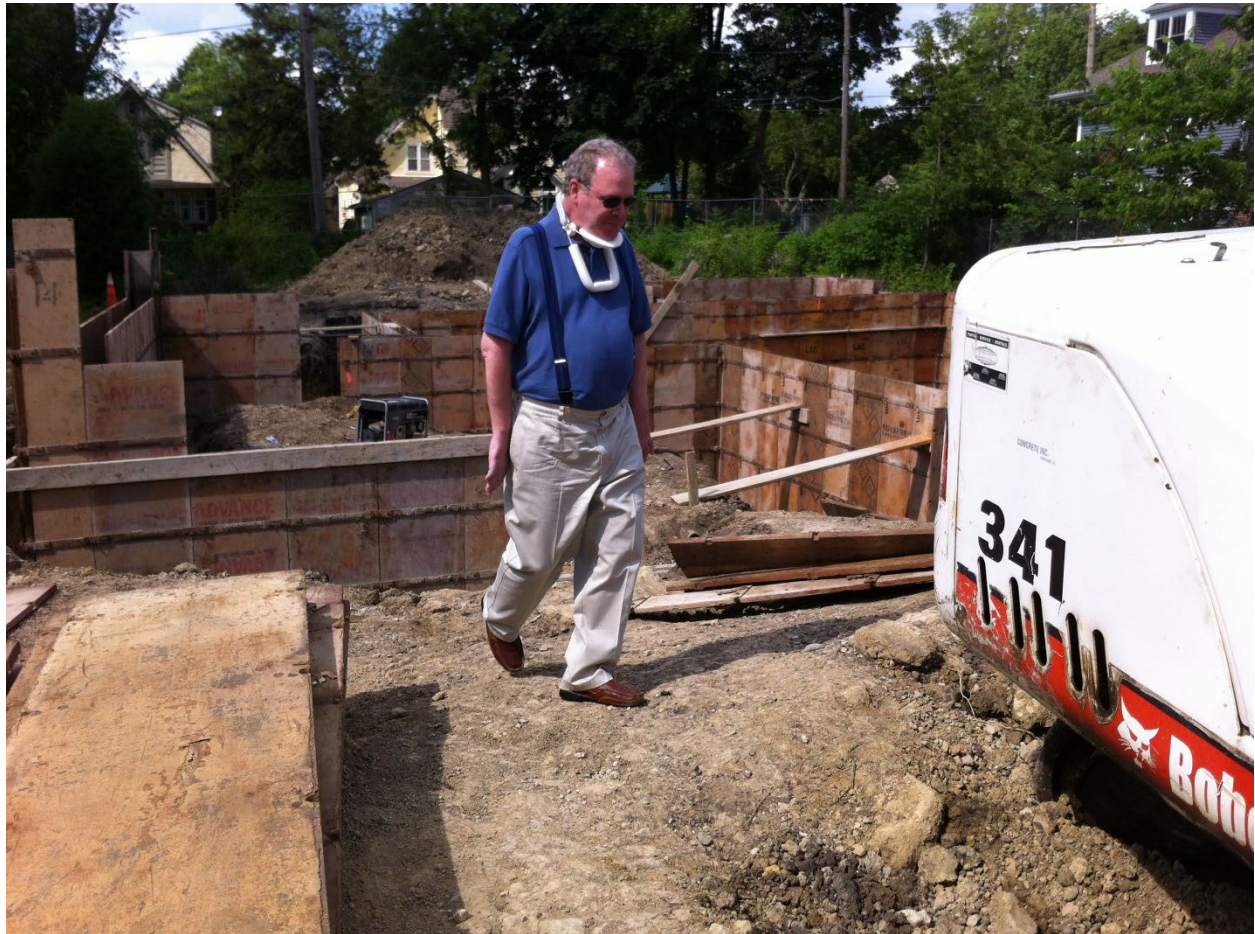
Photo 7; touring the construction site
