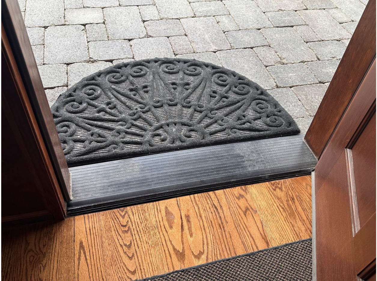
Photo 10; flush threshold looking out through the front door
